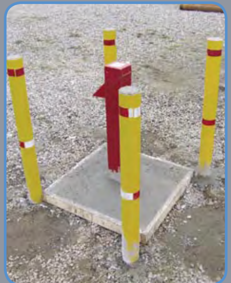
■ Finished observation well.
