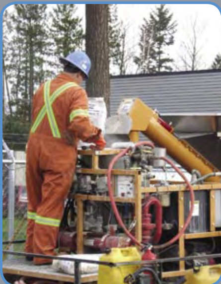
■ Grouting of bore hole.
