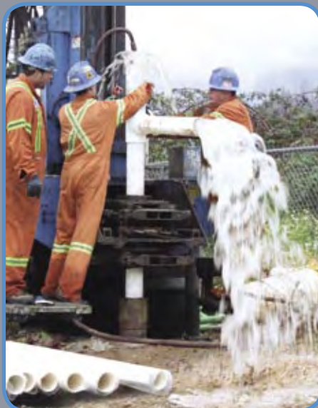
■ Well development in progress.
